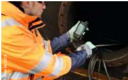
Entry into confined spaces/clearance measuring
